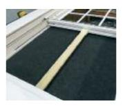
**7** Using the brace cut earlier push sash to upper position and place under sash.
