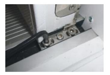
For the bottom track loosen allen bolts then adjust the middle bolt. This has a cam action that moves the door in and out.
