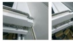
6 When fitting the sash you will notice that the flipper weather seal is inverted and catches on the plastic channel on the frame. To help ease the sash into position you will need a 1mm thick gauge of plastic laminate, or similar material, to slide between sash and frame.
