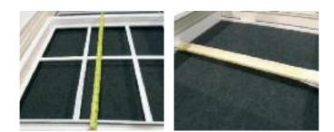
4 Measure the height of the sash from the top to bottom rail, work out the distance from bottom rail to cill, then cut a wooden brace and pad the brace at either end so as not to damage the sash or frame.
