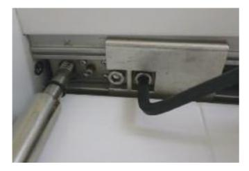
■ For the top track loosen allen bolts to move the hinge sliding the gear backwards or forwards to achieve the correct tolerance.
