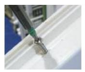
**3** Loosen off screws on the side of the sash but do not remove.
