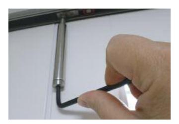
This allows the spindle of the hinge to be raised or lowered with an allen key that comes with your fitting box.
