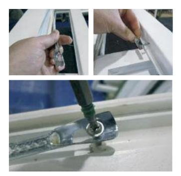
**5** Then position the sash between the parting bead and the external frame liner but leave the right hand side so that you can see the screw. Pull down the sash cord and hook it onto the screw and tighten. Using a 1mm gauge of plastic laminate, or similar material, as in item 6 (installing spring balance sashes) and slide the sash into place.
