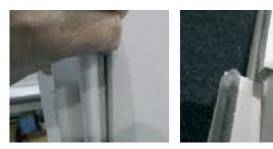
1 Remove right hand side of staff bead, this should be left partly unclipped, then remove right hand side of parting bead.
