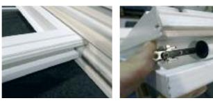
**5** Offer the top sash up to the frame, slotting the left hand spring groove on the sash over the left hand spring. Then place the right hand spring in the spring groove on the sash. Then replace the sash into the frame.
